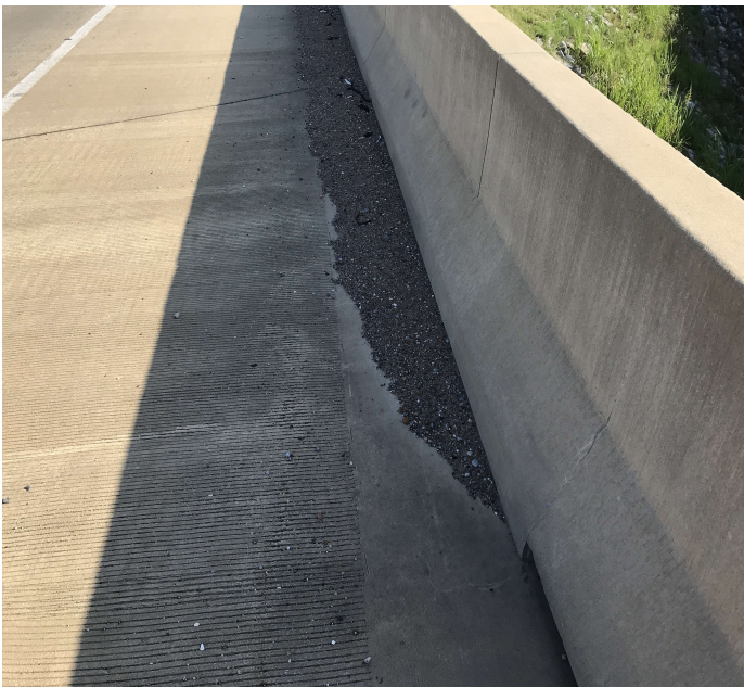
PHOTO 1 Description Gutters have debris in them.
