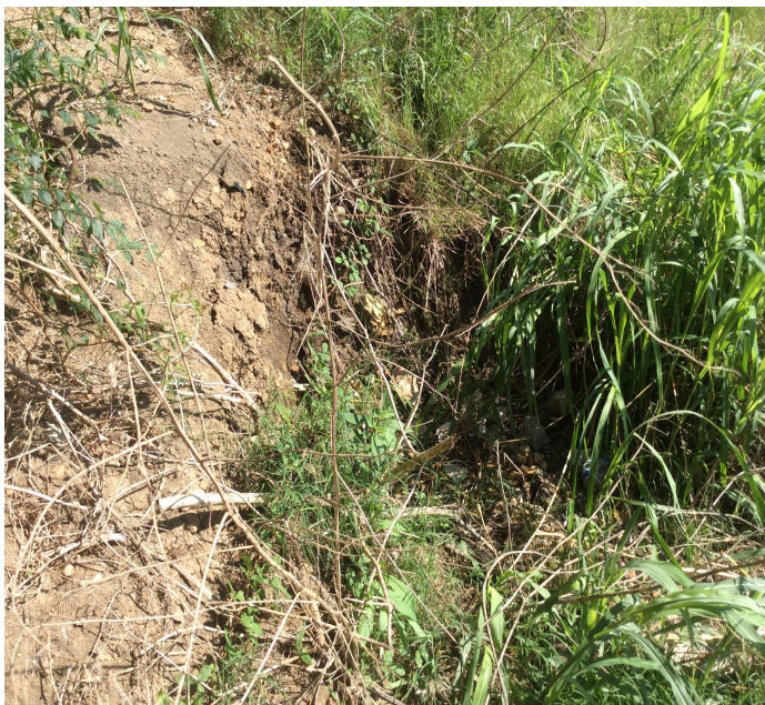
PHOTO 1 Description abutment 2 right side has eroded area up to 3' deep.
