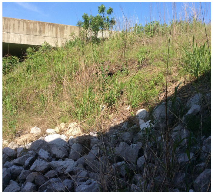
PHOTO 2 Description Slide north west side of bridge.
